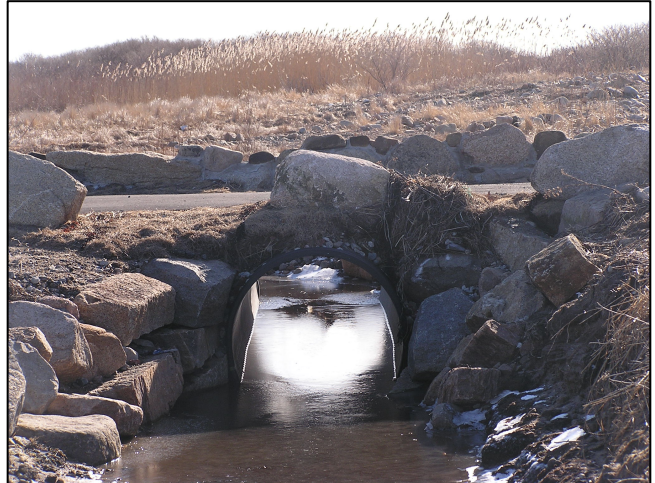
Culverts run under roads and allow water from the ocean to enter a marsh. Phragmites can be seen growing in the background.
