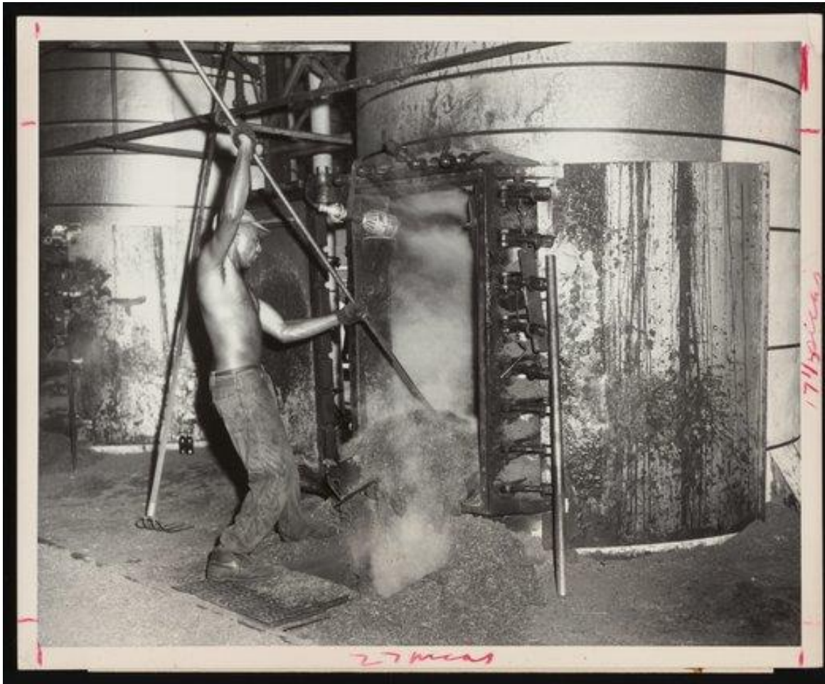
Hercules Incorporated. “Edward Newmans Clearing Extractor Tank at Hercules Brunswick Plant,” circa 1960. Photographs from the Records & Ephemera of Hercules Incorporated, Box 1, Folder 6. Science History Institute. Philadelphia. https://digital.sciencehistory.org/works/7h149q74m .
