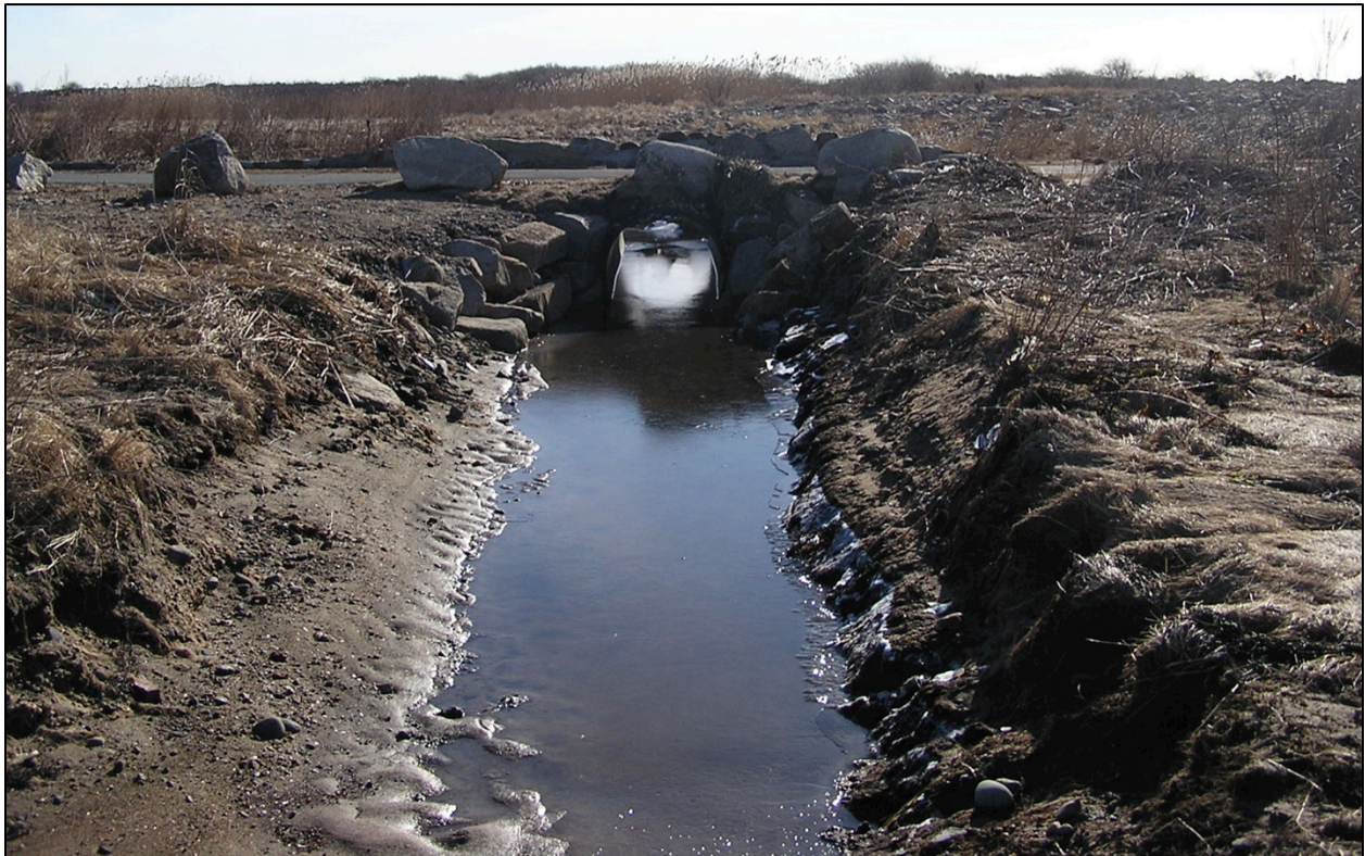
Figure 4: In December 2003, scientists dug a channel, which provided fish passage to a culvert under the road. The restoration brought back water flow between upstream and downstream of the tidal restriction.
