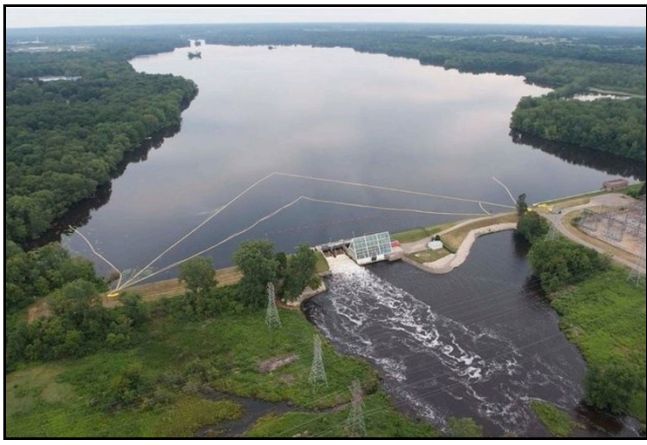
A reservoir created by a dam along the Kalamazoo River. When water flows into the reservoir it slows, potentially letting some of the total suspended solids settle to the bottom.
