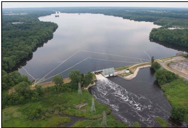
A reservoir created by a dam along the Kalamazoo River. When water flows into the reservoir it slows, potentially letting some of the total suspended solids settle to the bottom.
